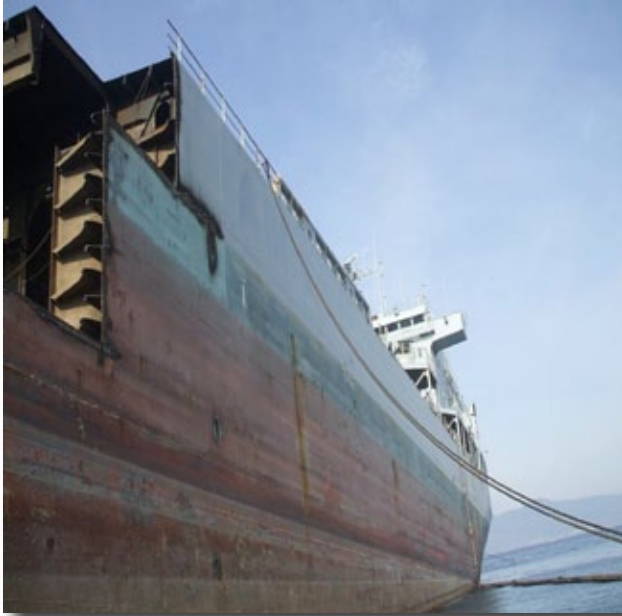
Early stages of Dismantling
