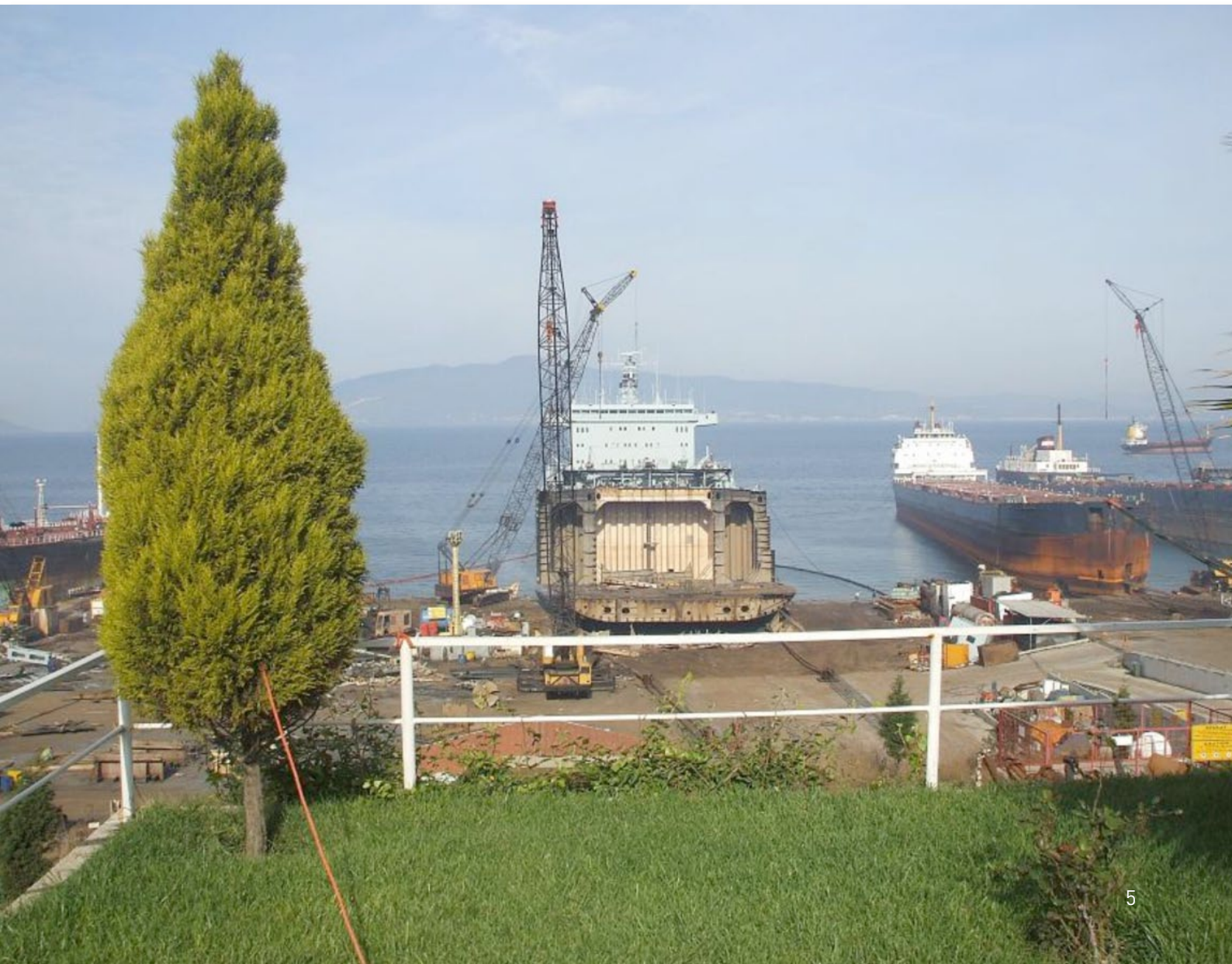
Dismantling of Ex RFA Oakleaf
