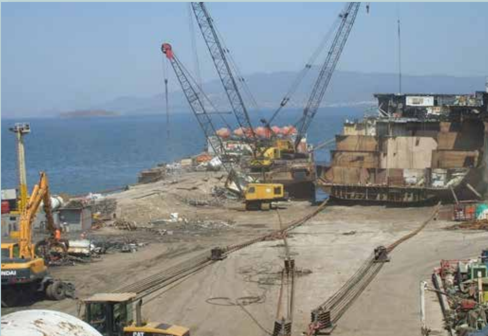
Progress of works 06/06/2013. The remaining part of the keel is winched on to the dry slip way
