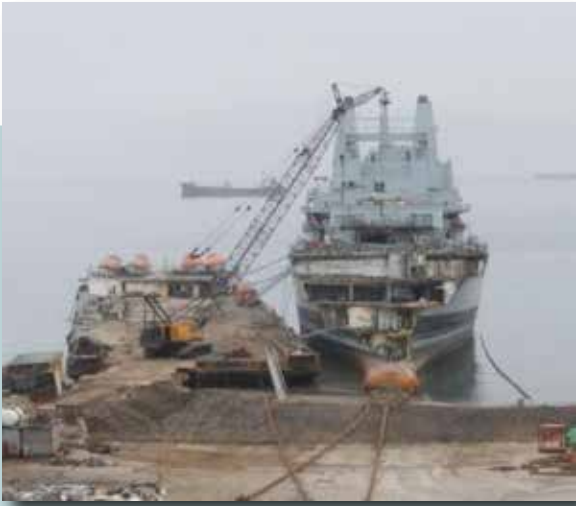
Dismantling and progress of works dated 17/04/2013
