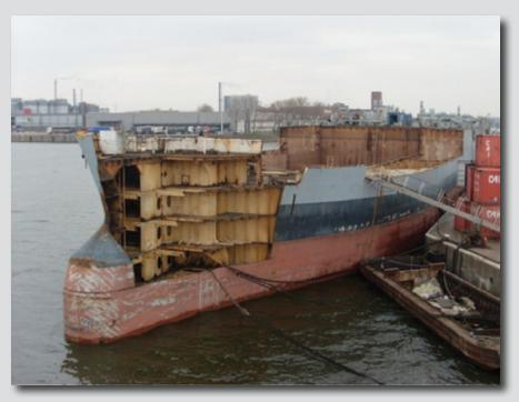
3 photos showing superstructure completely removed, the Engine room opened up and the first "layer" of the ballast/diesel tanks almost all removed
