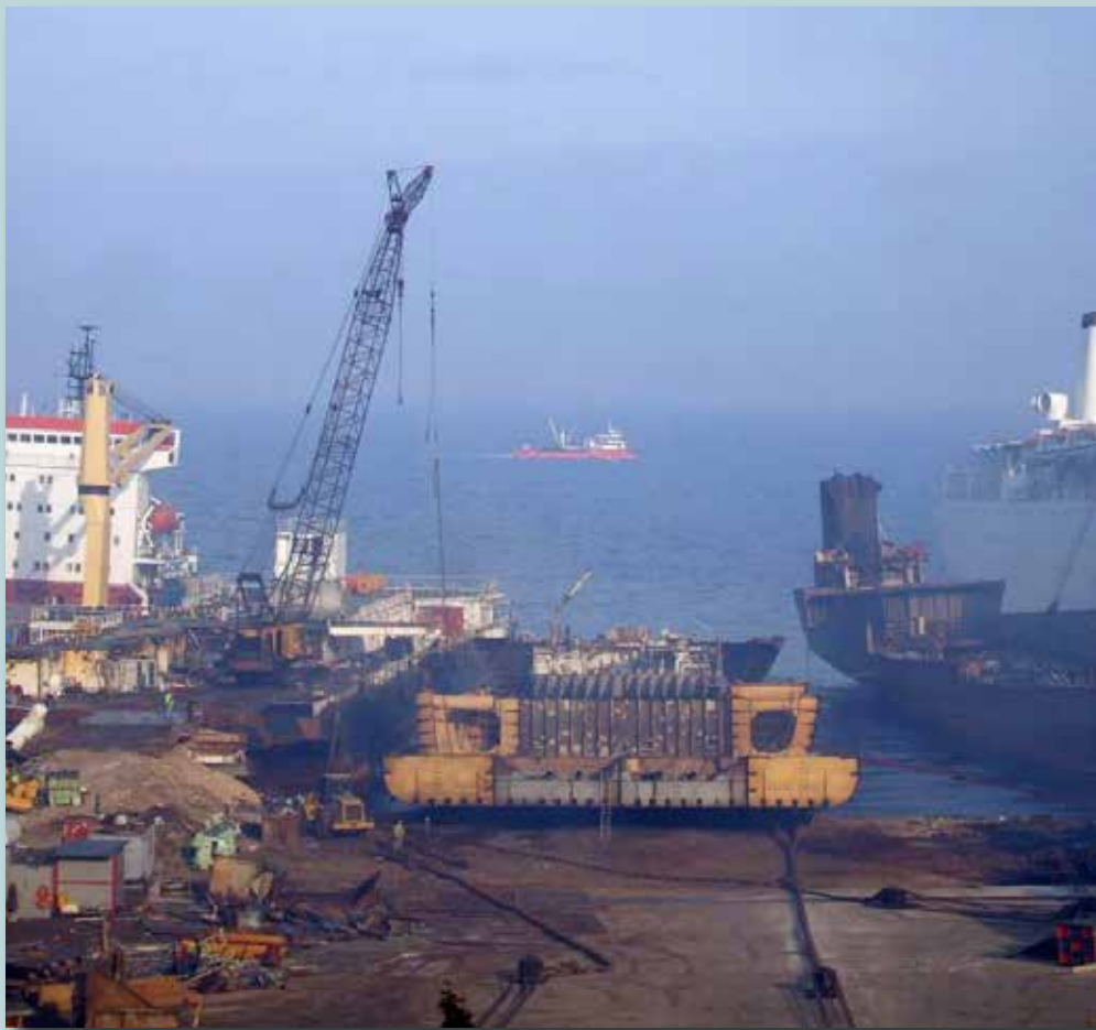
Ex-RFA Bayleaf 28/11/2012 Final dismantling of Pump and Engine Room
