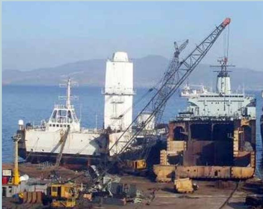
Progress of works 30/10/12 Dismantling of bow, fore peak, deep tanks
